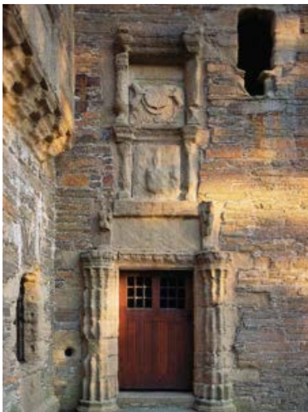
Figure 2 Carved Stones are often vulnerable to weathering and environmental erosion: external doorway at Earl's Palace, Kirkwall.
