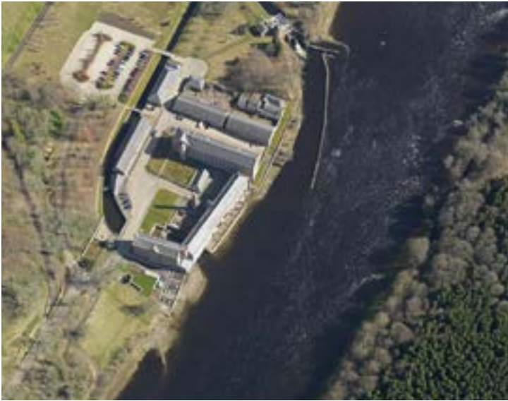
Stanley Mills hydroelectric power station © HES
