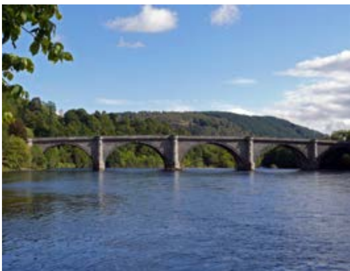
Telford's Bridge in Dunkeld © Perth and Kinross Heritage Trust
