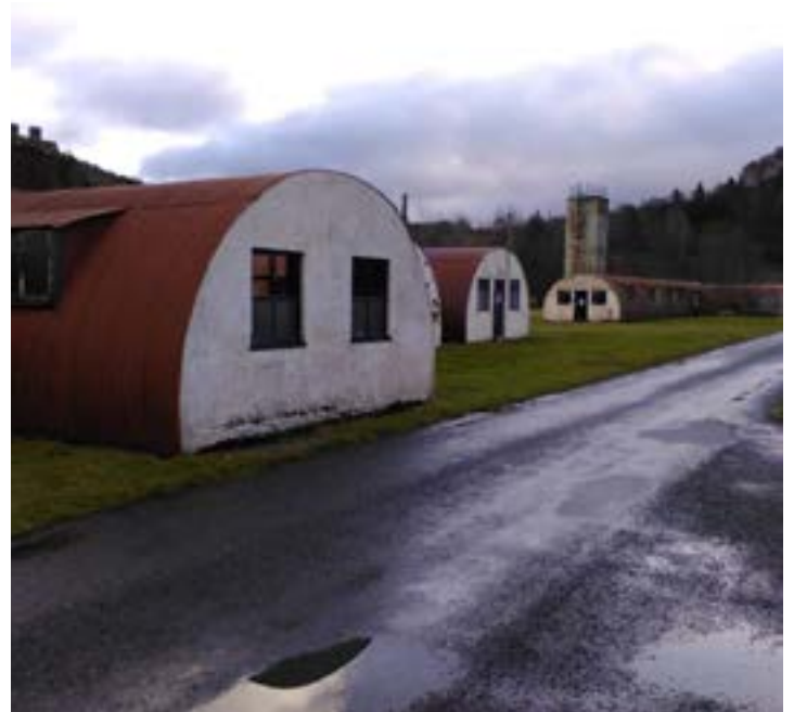
Buildings at Cultybraggan POW camp © Perth and Kinross Heritage Trust
