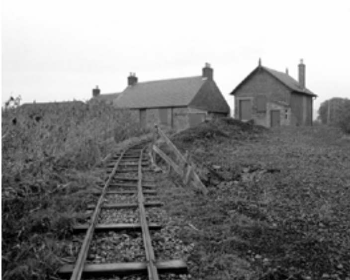
Remains of railway line at Cairnie Pier © HES
