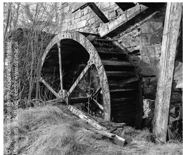
Figure 7. The waterwheel at Craig Mill, South Lanarkshire, a 19th-century replacement of an earlier wheel.
