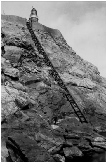
Figure 10: The access to some lighthouses was complex and dangerous, such as at Muckle Flugga, Unst, Shetland. The light railway was used to take supplies from vessels up the cliff. The permanent light was established on the most northerly rock of Scotland, when it was lit on 1 st January 1858, © RCAHMS DP049358.
