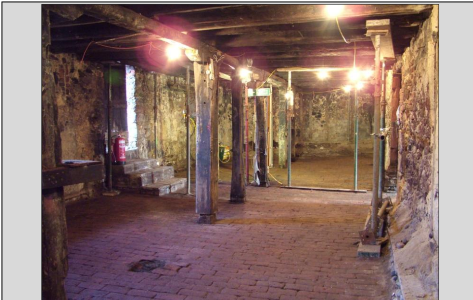
Figure 18: Re-used ship timbers from MacArthur's store in Dunbar. The deck beams from a likely 18 th century coastal trader offer rare insights into ship timber assemblages in the Scottish vernacular context and the possibilities that abound to study the tangible remains of the Scottish merchant marine, © Headland Archaeology.
