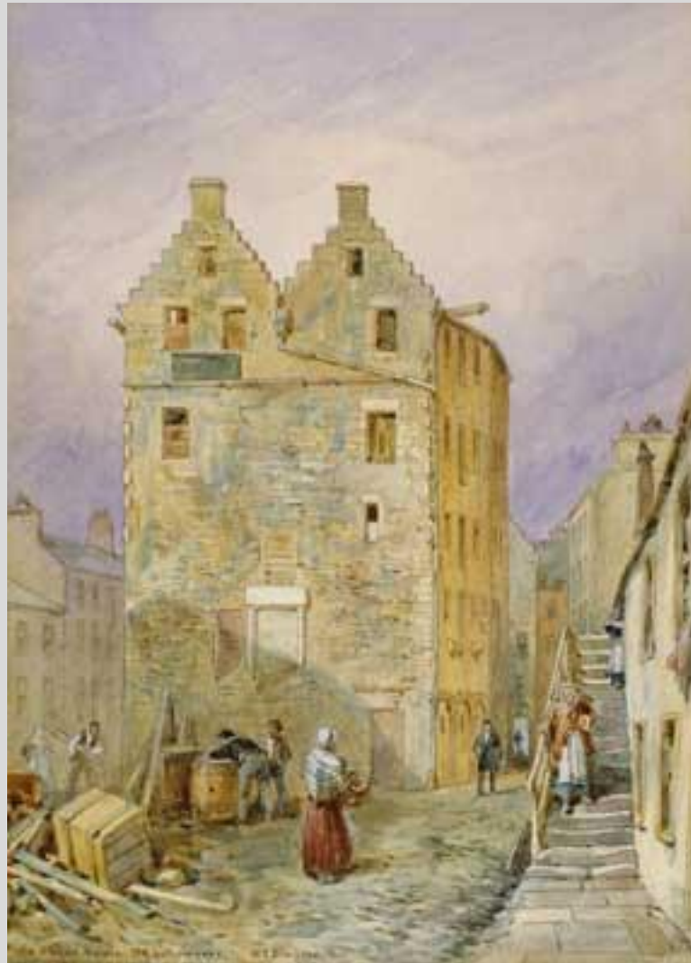
Figure 10: William Simpson's painting 'Old Sugar House, 138 Gallowgate, circa 1845' indicates the character of the sugar processing factories which were constructed in the 17 th century in association with Glasgow's emerging colonial economy © Culture and Sport Glasgow (Museums): www.glasgowlife.org/museums
