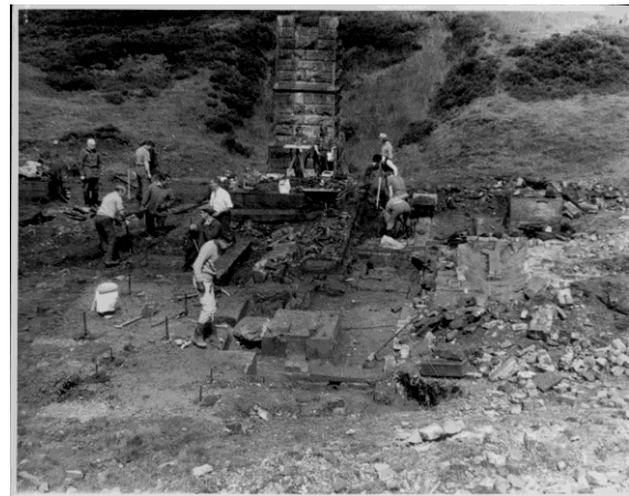
Figure 5: The image shows the Glasgow University Summer School excavations in the 1970s conducted at Bay Mine, Wanlockhead, site of the first Watt engine built by George Symington. The excavations revealed foundations of engine- and boiler-houses. Reproduced by kind permission of the Wanlockhead Museum Trust: www.leadminingmuseum.co.uk .
