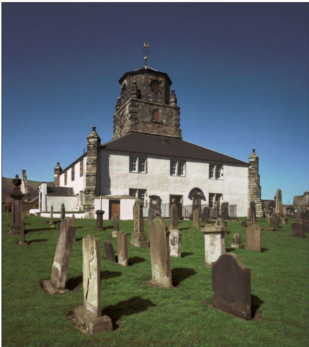
Figure 28: Burntisland church. An early post-Reformation structure built to accommodate a central pulpit with a square 'nave' surrounding the central focus. Recently restored, the building can accommodate a large congregation using galleries as well as stalls around all four side 'aisles', © RCAHMS
