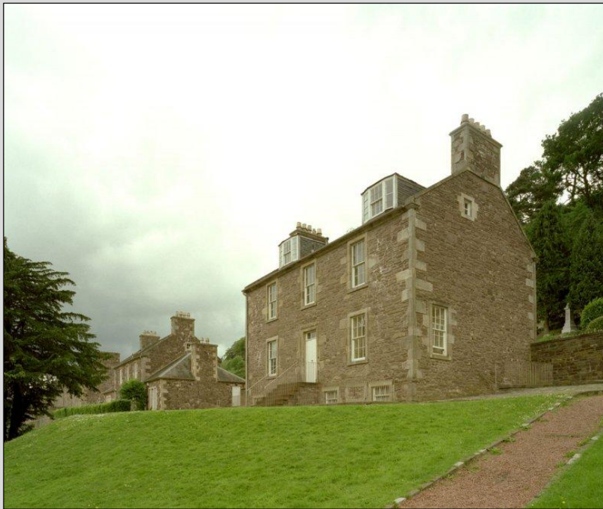
Figure 8: Owen’s improved settlement nevertheless retained class divides, and in fact used the principles of surveillance of the workers to enforce their desired patterns of behaviour. Owen’s own house was centrally positioned with a view not only of the mills but also of the residential streets and the institutional buildings, and controlling the main routes of communication between places of residence, work and leisure in the village, ©RCAHMS.
